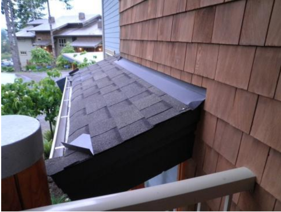
Metal flashing
