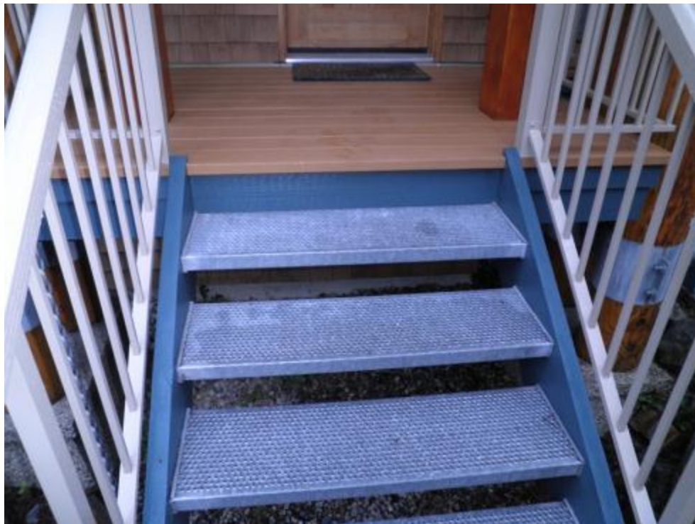
External stairs (galvanized metal treads)
