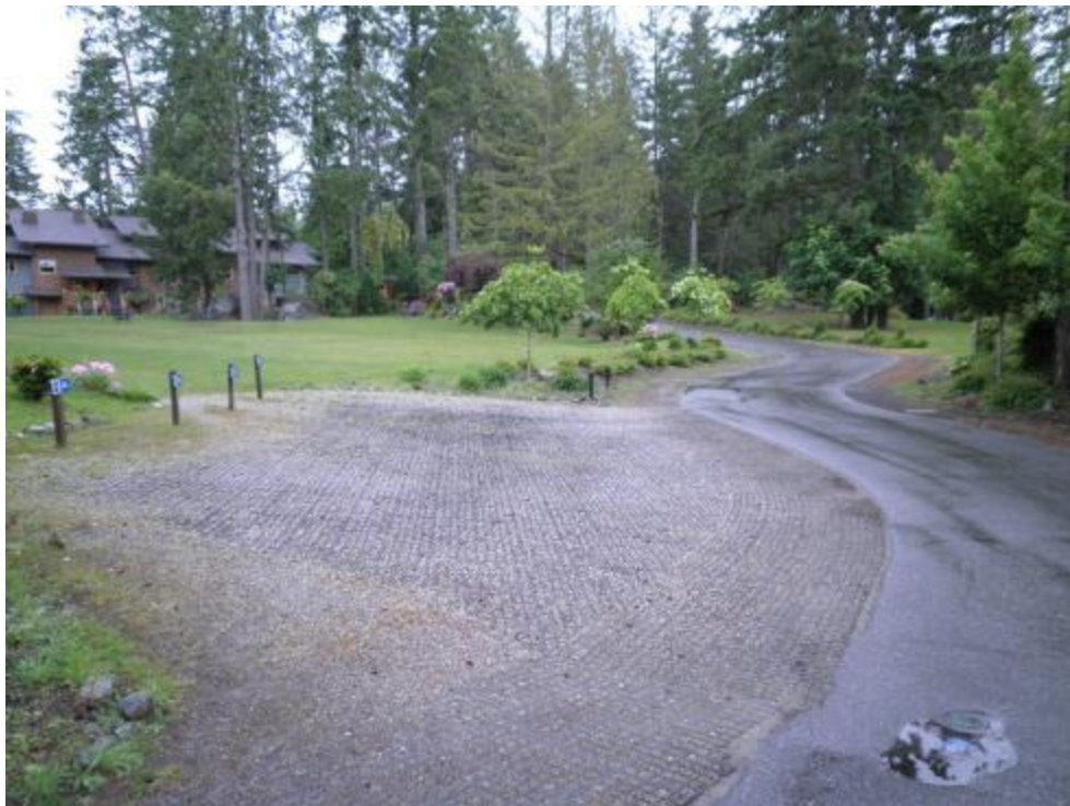
Eco-grid paving and parking area
