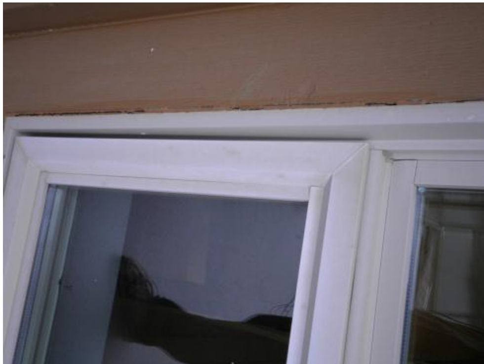
Caulking with signs of deterioration
