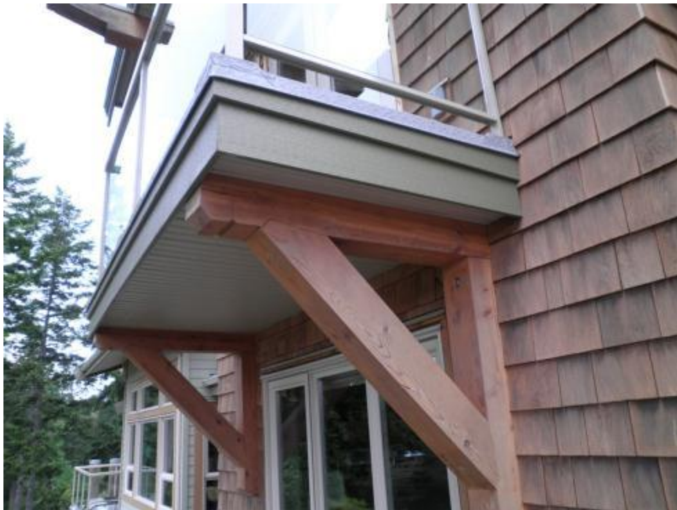
Wooden balcony covered with vinyl membrane
