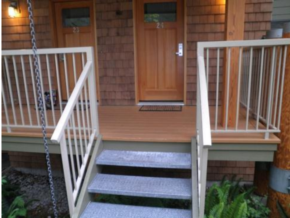
External stairs (galvanized metal treads)
