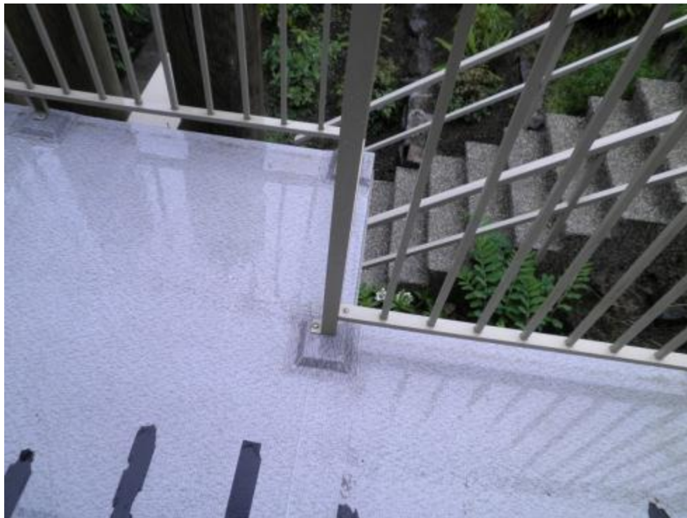
Vinyl membrane deck flooring
