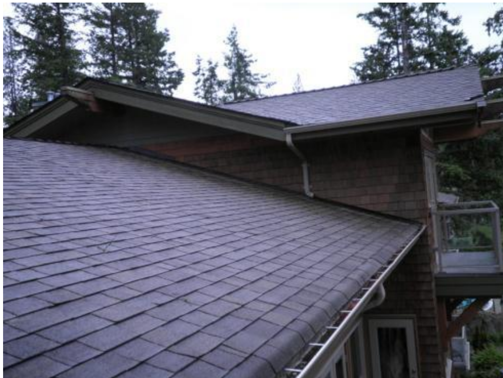
Fibreglass reinforced asphalt shingles
