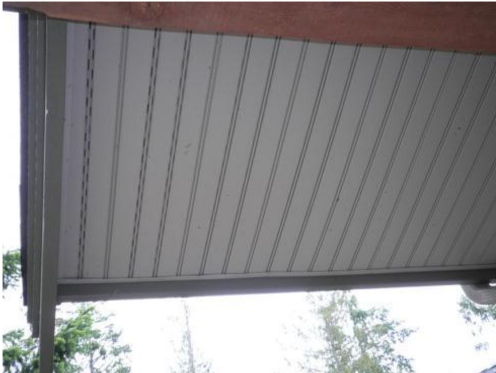
Exterior vented vinyl soffits
