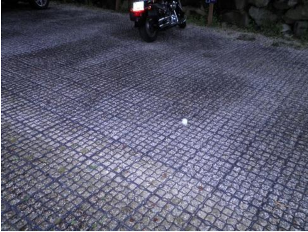
Eco-grid paving and parking area
