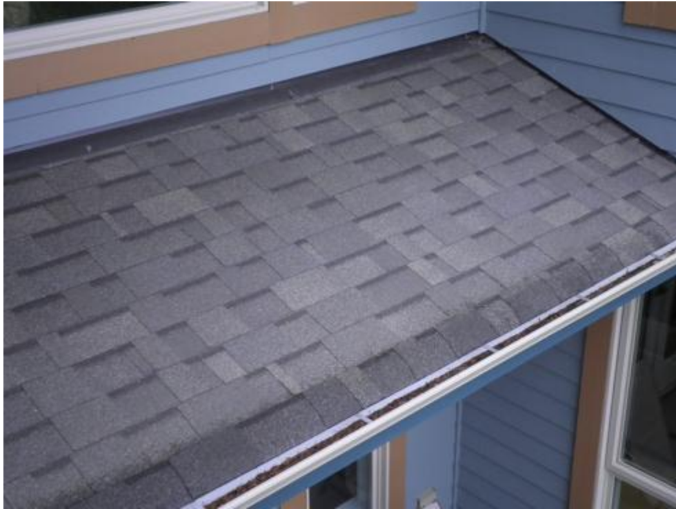
Fibreglass reinforced asphalt shingles
