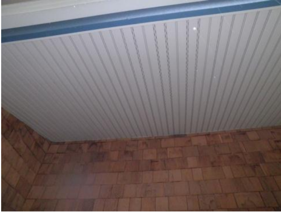
Exterior vented vinyl soffits
