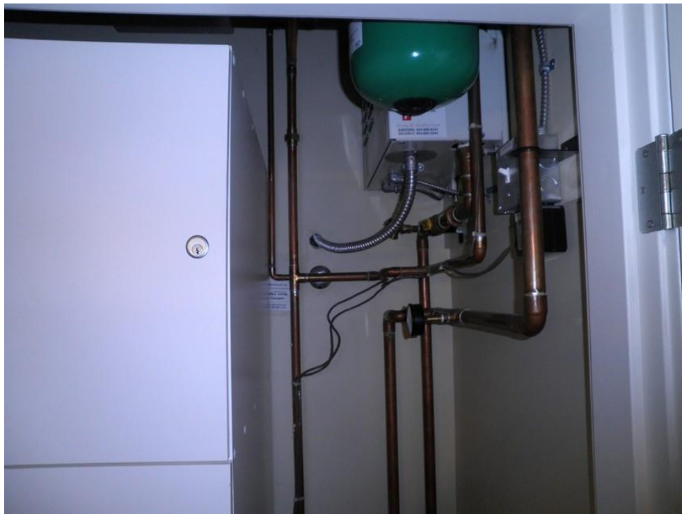
Boiler(white) setup with expansion tank(green)
