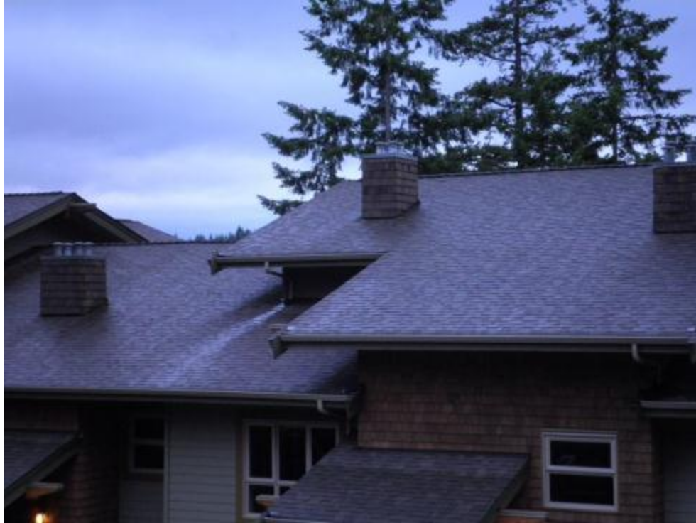
Cedar shingle clad vent chimneys
