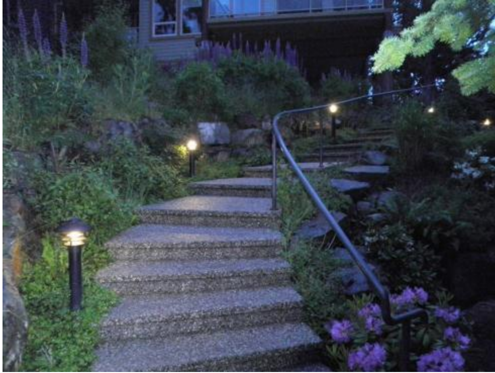
External stairs (concrete aggregate)
