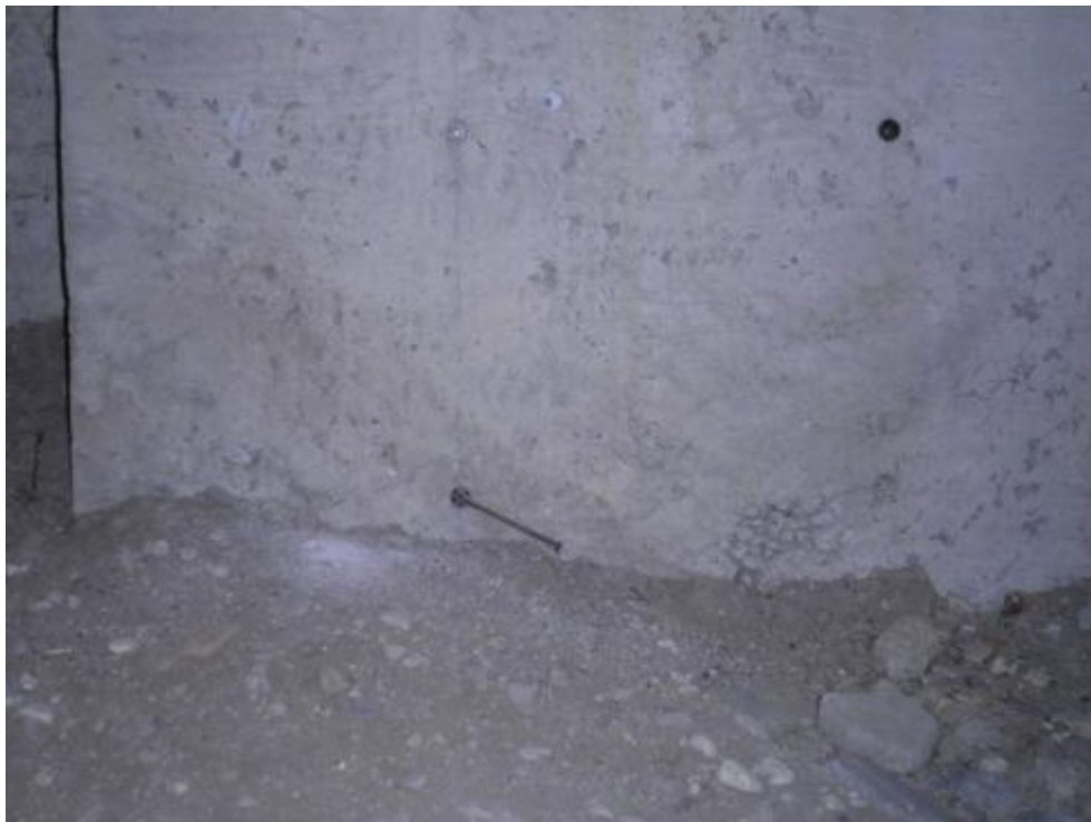
Exposed rebar in foundation walls
