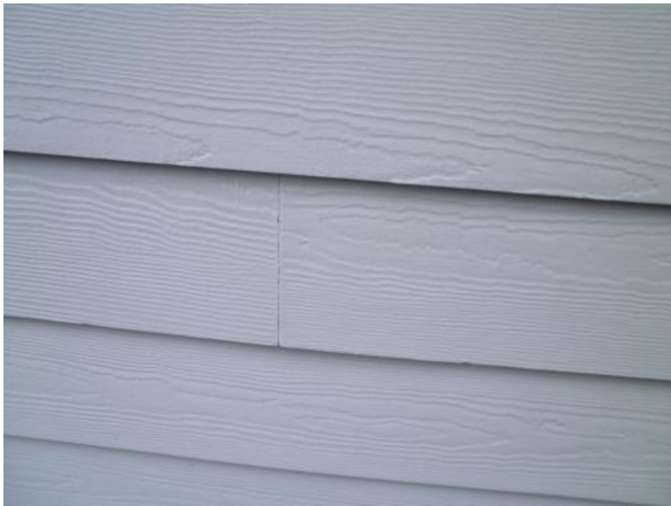
Cement board siding
