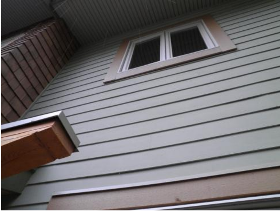
Cement board siding
