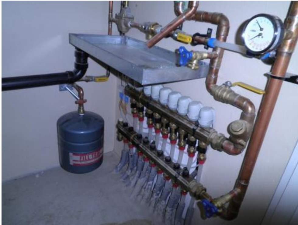
In-floor radiant heating system
