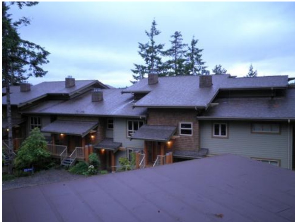
Cedar shingle clad vent chimneys
