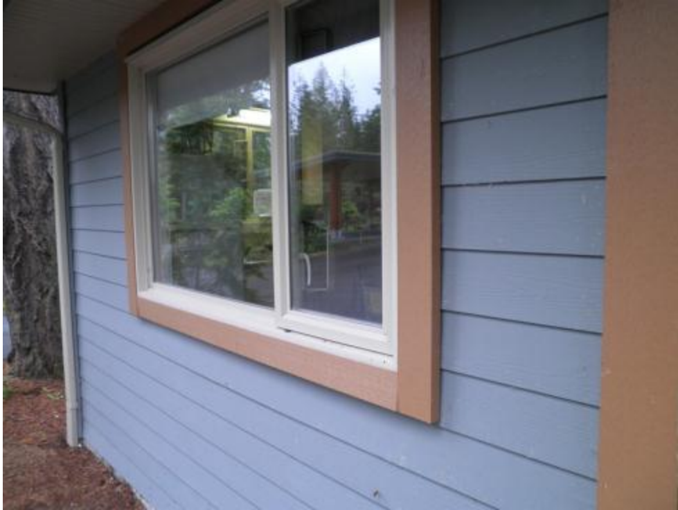
Exterior paint (cement board siding)
