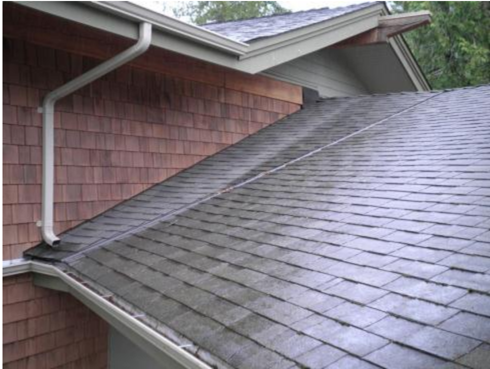
Gutters and downspouts
