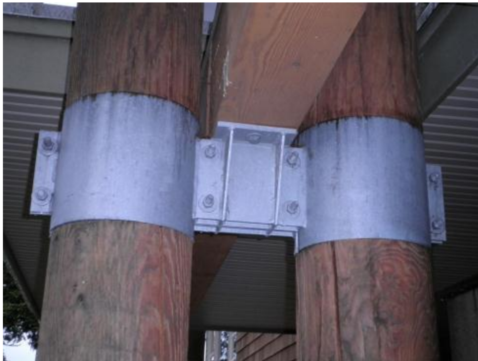
Wooden support columns needing refinishing
