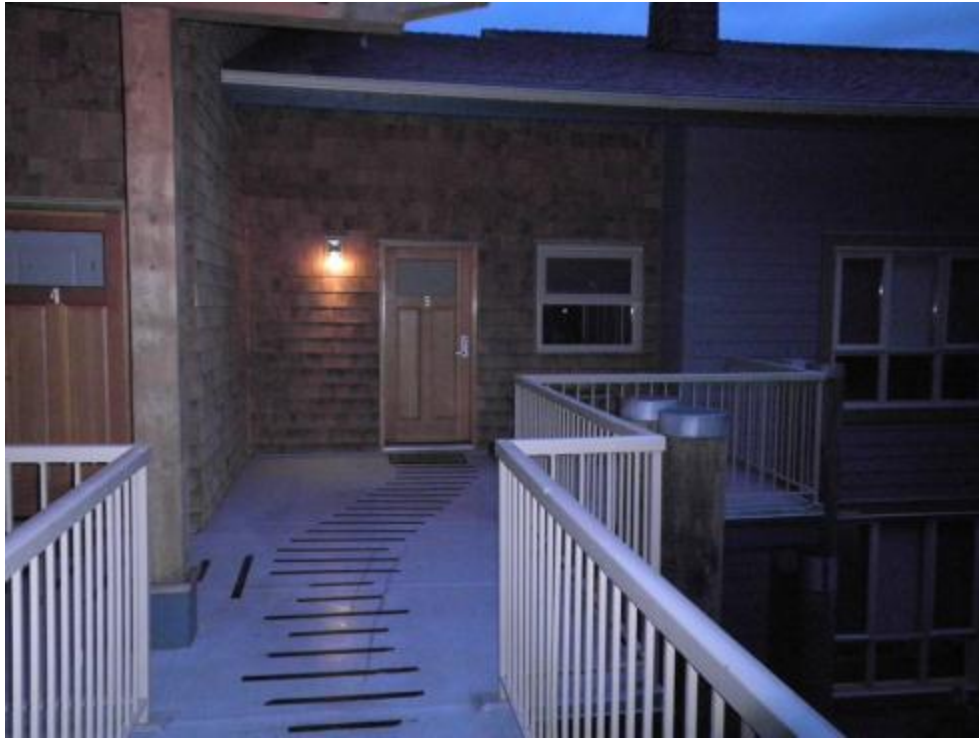
Vinyl membrane deck flooring
